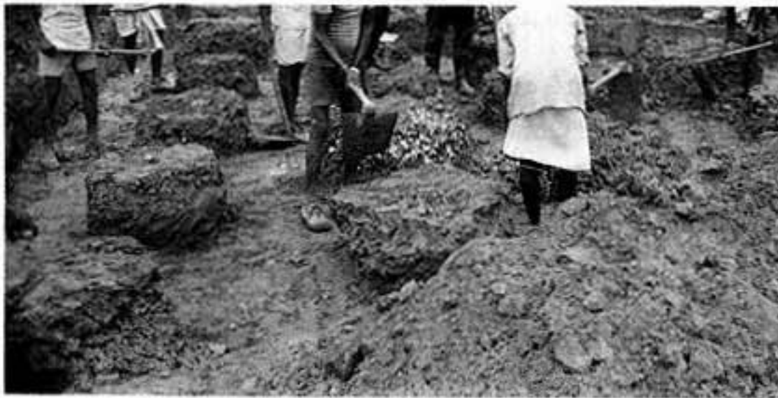
Fig. 13 View of Exposed Gravel Piles
